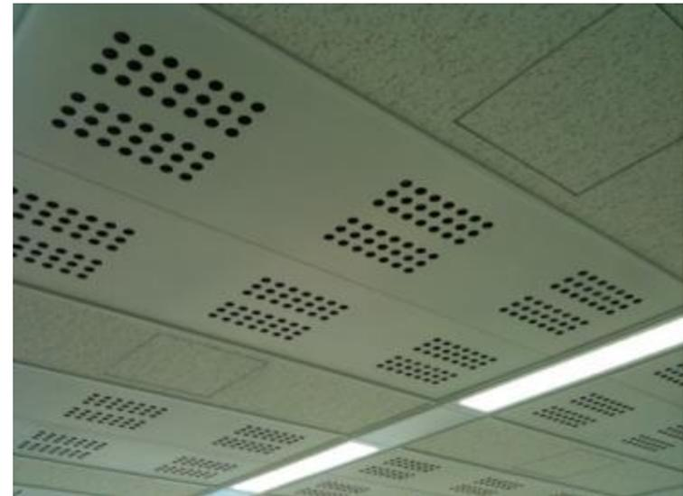
Radiant panels are occupied 45% of ceiling area
