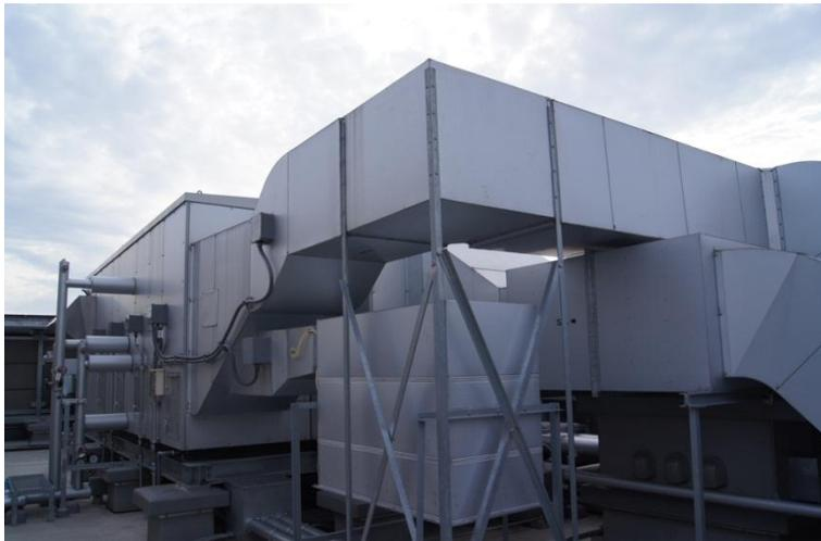
Desiccant dehumidifier is installed as air handling unit for supply fresh air . Exhaust heat from heat pump is utilized as recovery heat for desiccant rotor.
