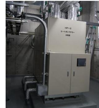
Water Source Heat Pump (120kW)
