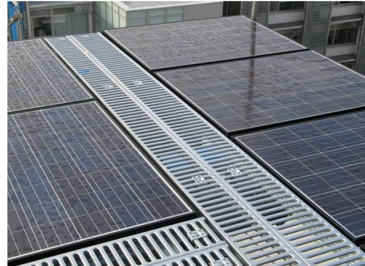
Thin type of multicrystalline Si PV of 30kW(=300m<sup>2</sup>) is installed. The total electricity production is expected to about 150GJ/a. in specific and 375GJ/a in primary energy.
